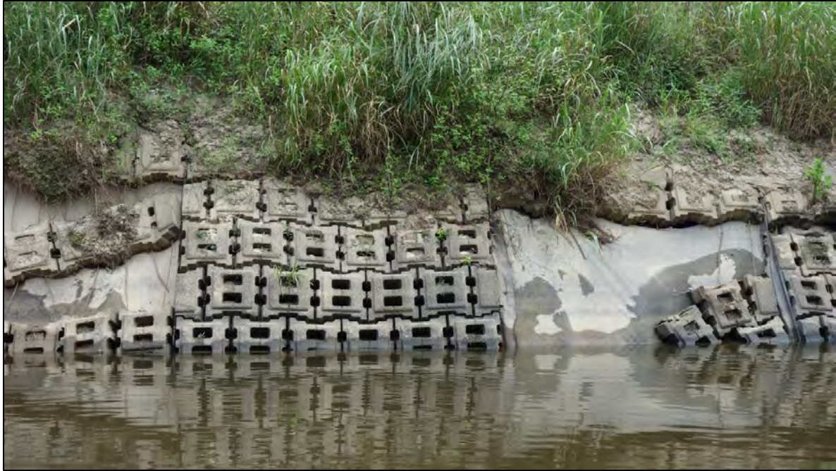
Figure 4-2. 2011 project in state of degradation (photo: USACE site visit 2020).
