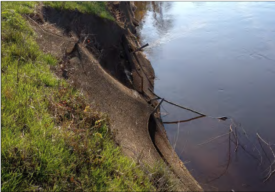
Figure 5. Riverbank erosion, 2011 – Pre-Remediation
