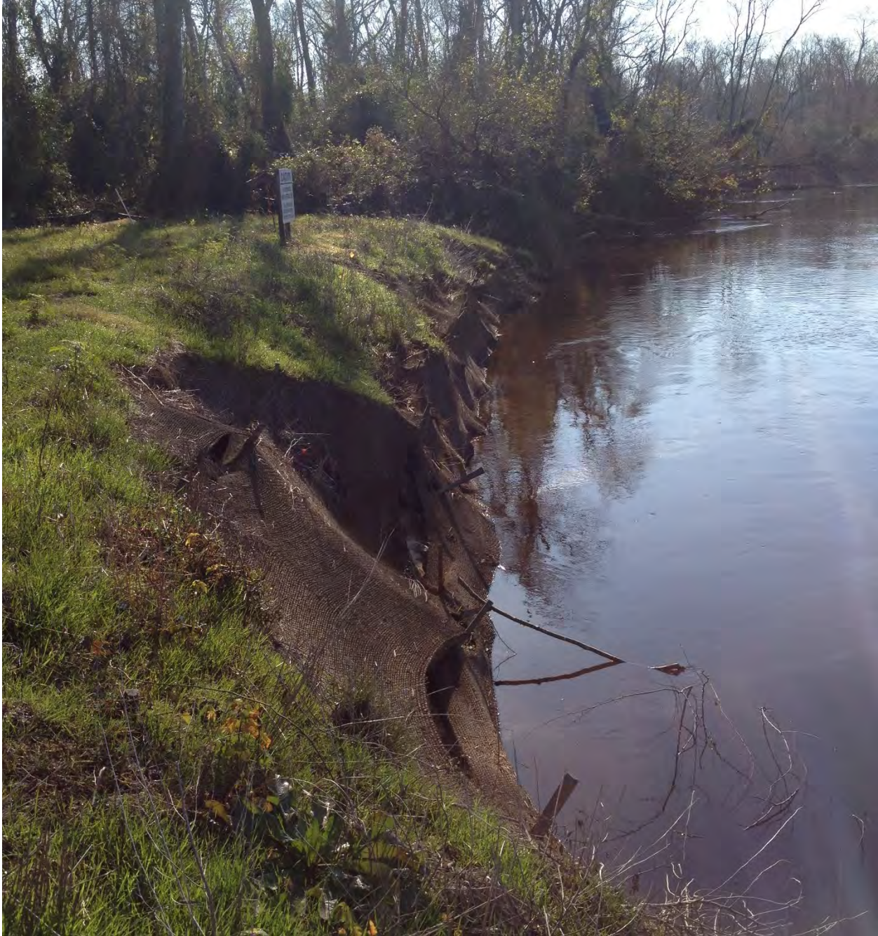
Figure 4-1. Riverbank erosion prior to 2011 project.
